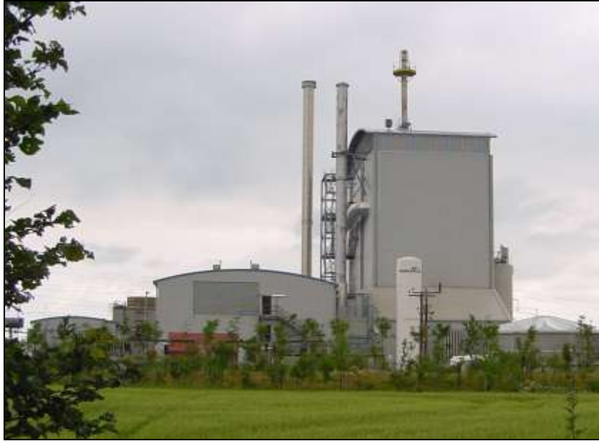
Figure 25 The ARBRE plant in June 2001
