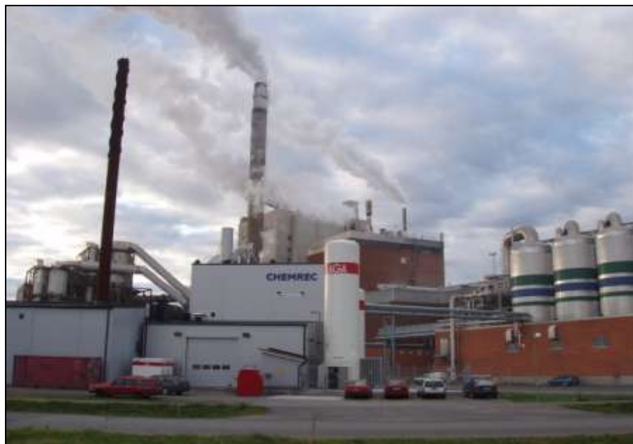
Figure 31 Pressurised development plant DP-1 at Kappa Kraftliner pulp mill, Piteå
