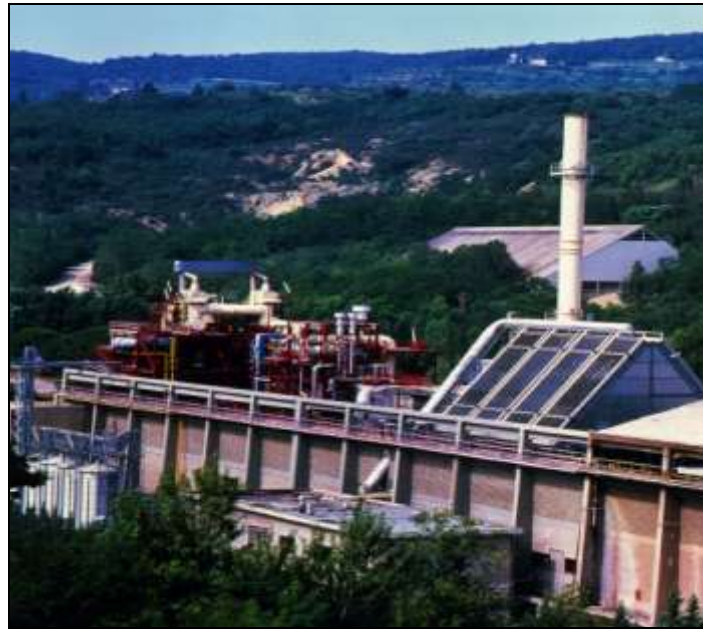
Figure 14 TPS/Ansaldo RDF gasification plant in Grève, Italy
