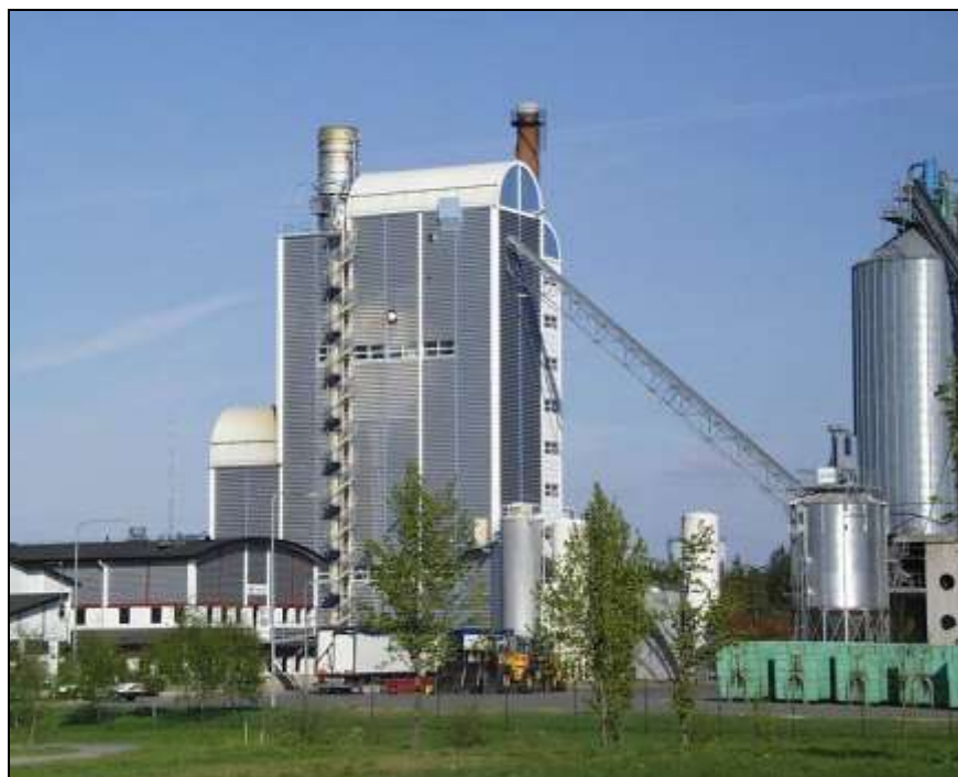
Figure 16 World's first complete biomass-fuelled IGCC power plant at Värnamo
